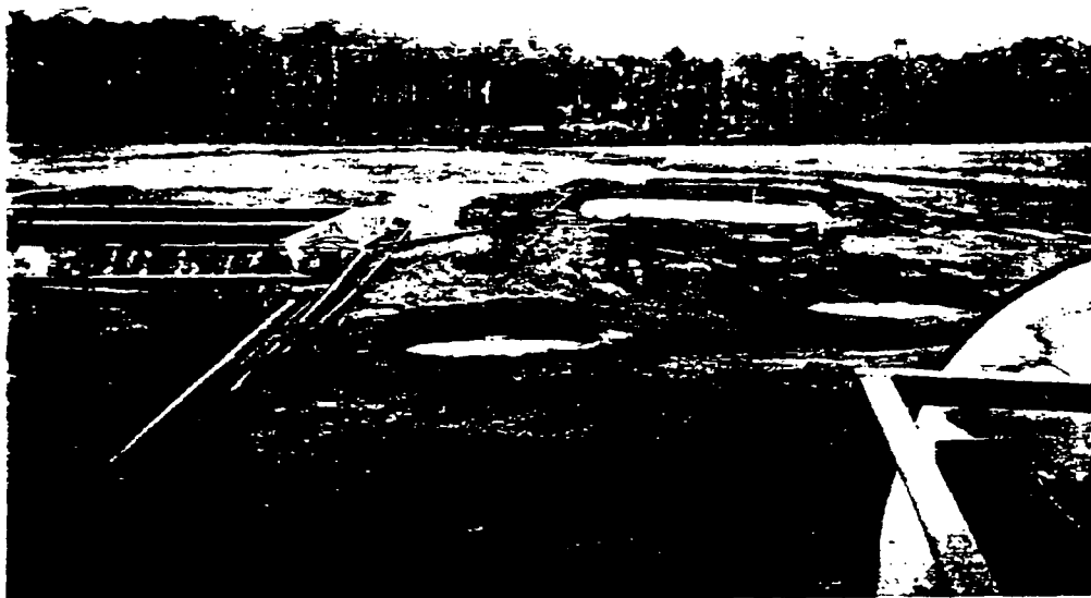
Photo J-26: Produced water separation pits at Sacha Central Production Station.
