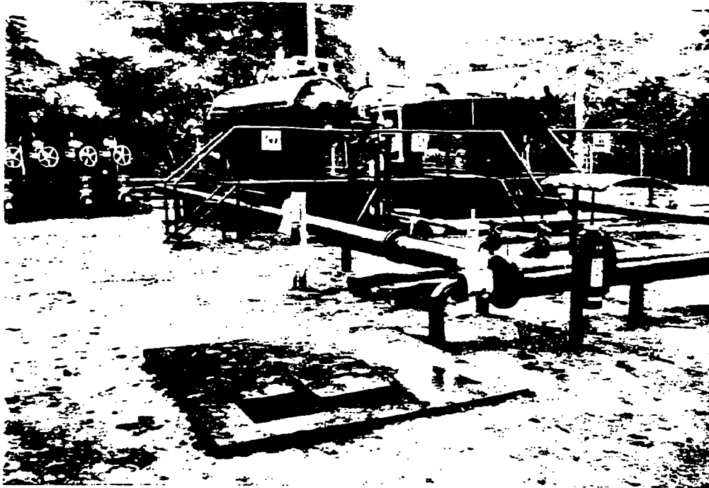
Photo J-15: Separators and process area sump at the Atacapi Production Station. Spills are typically covered with sand.
