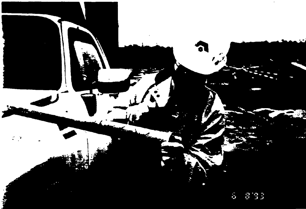
Photo 8-2 A slotted interval of 0.3 meters was cut in the PVC prior to installing the piezometer.
