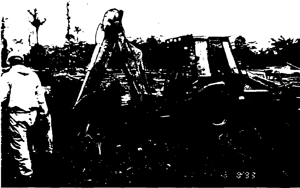
Photo 8-1 Backhoe used to excavate test pits at Shushufindi Field.
